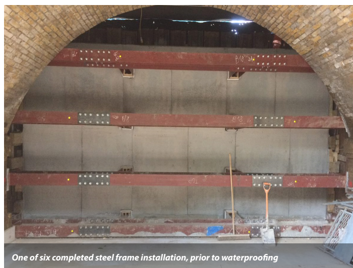
A 'no fines' concrete wall was constructed at the back of the steel frames to retain the embankment
