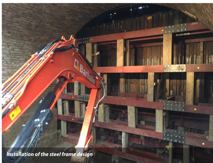
A 'no fines' concrete wall was constructed at the back of the steel frames to retain the embankment
