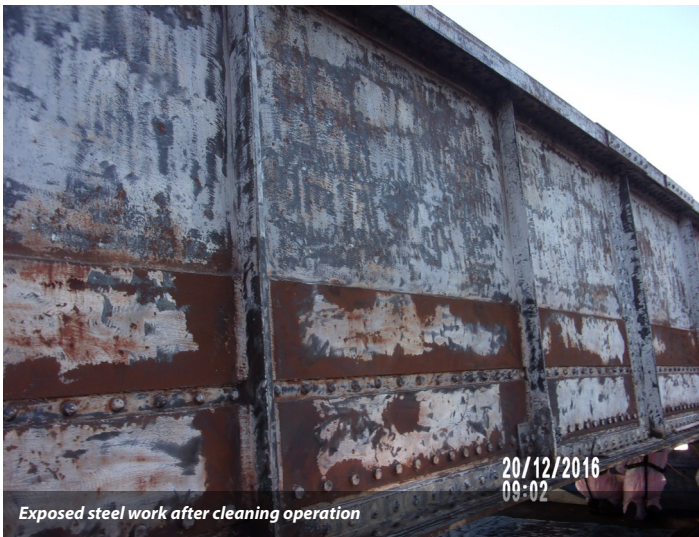
Underside deck conditions pre-work
