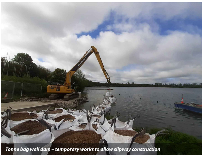
RC Concrete slipway construction – temporary dam wall installed and in use
