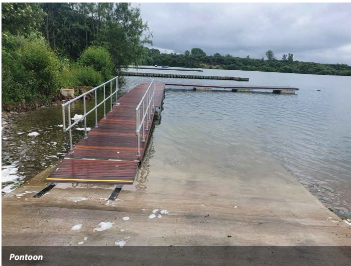
Concrete slipway and pontoon
