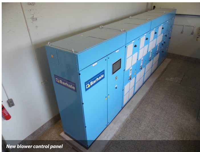
New blowers, blower house 1
