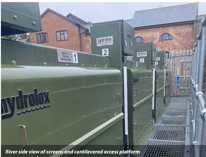
Porta-dam in position
