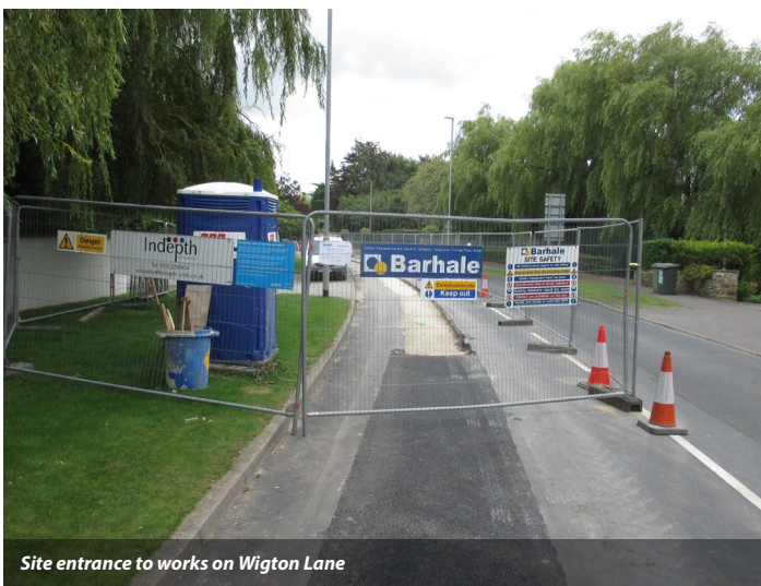
Trench planed off in preparation for excavation
