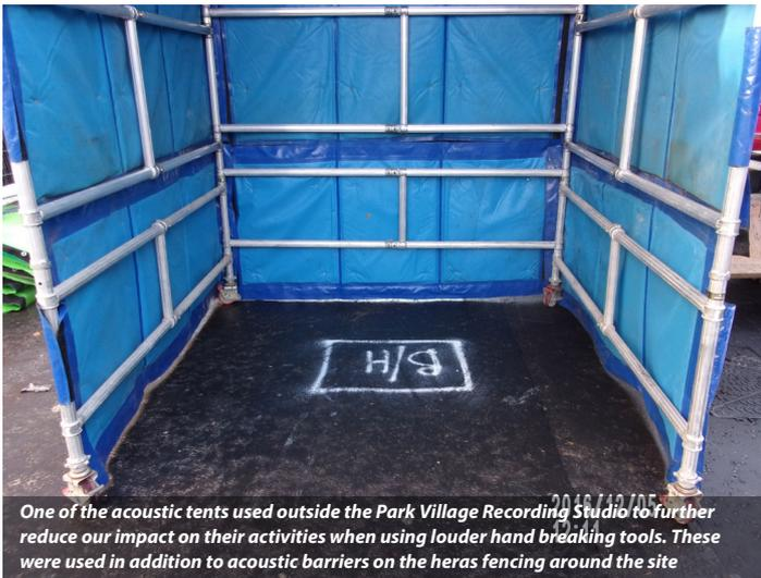
One of the acoustic tents used outside the Park Village Recording Studio to further reduce our impact on their activities when using louder hand breaking tools. These were used in addition to acoustic barriers on the heras fencing around the site
