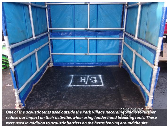
One of the acoustic tents used outside the Park Village Recording Studio to further reduce our impact on their activities when using louder hand breaking tools. These were used in addition to acoustic barriers on the heras fencing around the site
