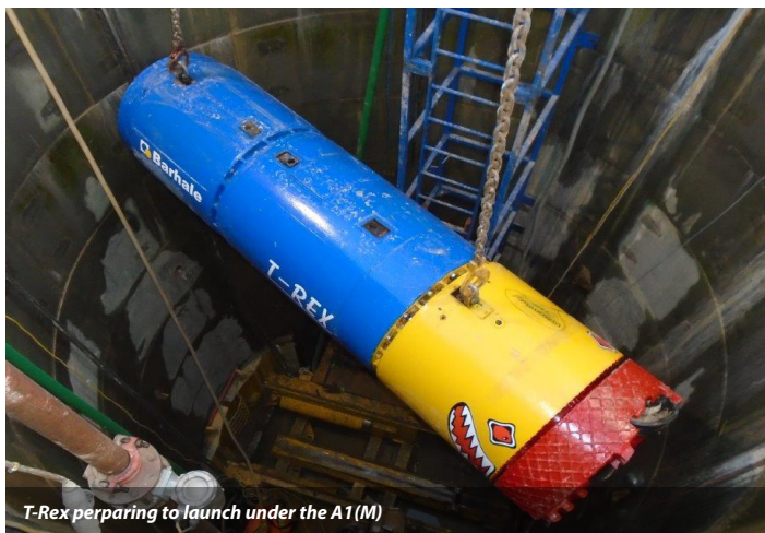
Directional drilling was utilised for 800m
