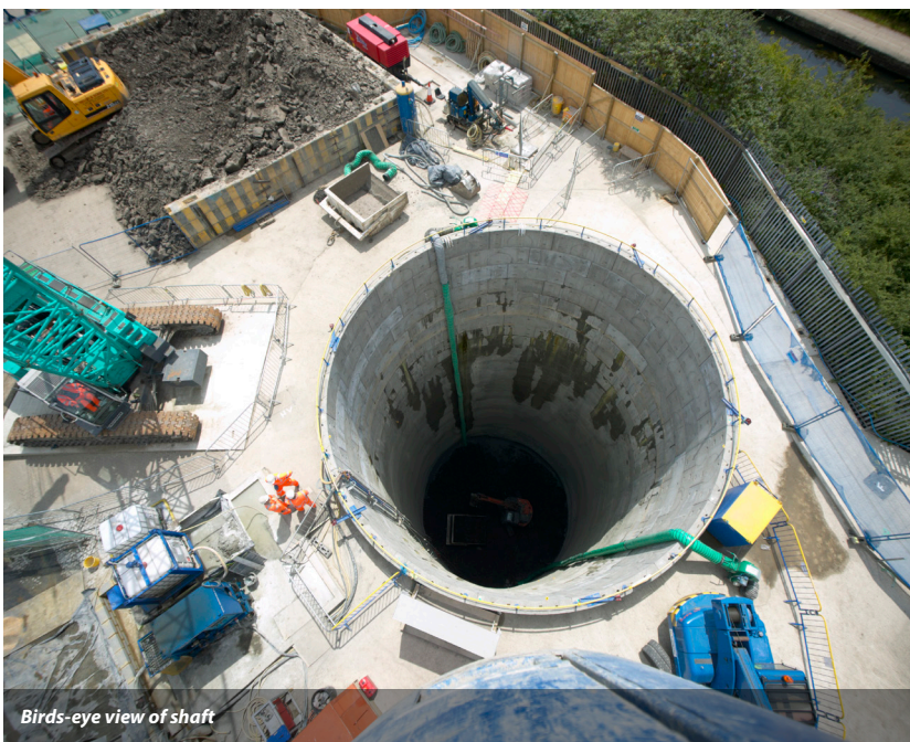
Excavation of shaft
