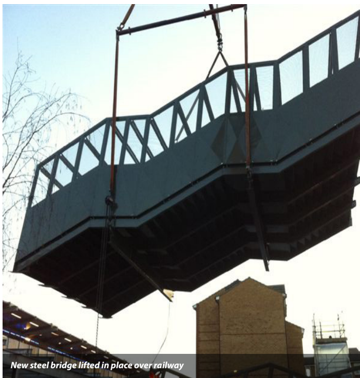
Steel structure to form walkway from the station platform
