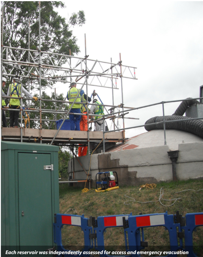
Temporary tanks supported the out of service reservoirs
