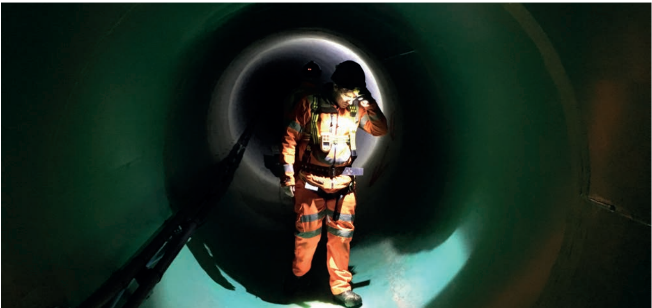
Above: Inspecting the Thames Water Ring Main
