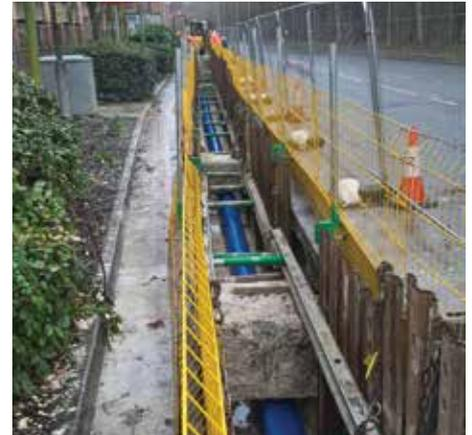
The team excavated 487m of water main trench, 418m of electrical trench and 100m of gas main trench
