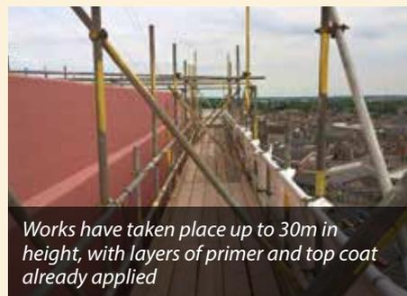
Works have taken place up to 30m in height, with layers of primer and top coat already applied
