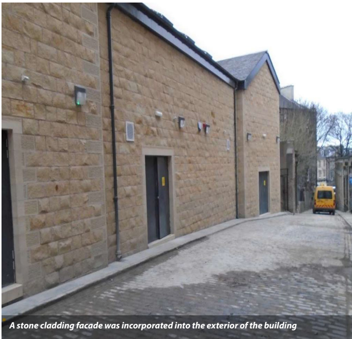
Reclaimed cobblestones were installed by specialist operatives
