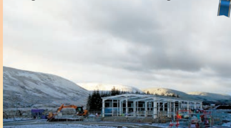
Glenglass Substation, Scotland Region
