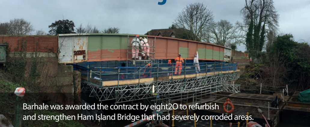
Quality inspection check between coating application
