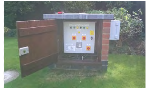
Hatch during refurbishment.
