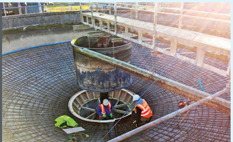
The photograph shows the carpenters putting the final touches to the formwork in preparation for the concrete pour scheduled for the following day.
