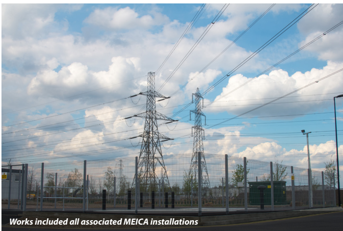
New pumping station - gravity sewers
