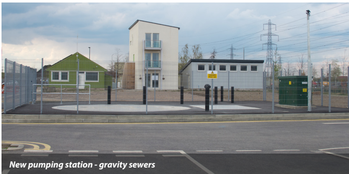
Completed pumping station compound
