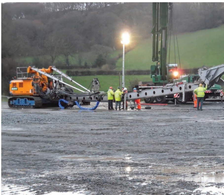
▲ Piling Rig being assembled before installing piles for launch Cofferdam
