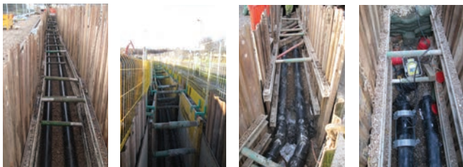
▲ Laying in carriageway ▲ Laying in verge ▲ Electrofusion joints and services ▲ Electrofusion jointing
