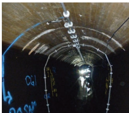
▲ Installed Shape Arrays inside the EVA
