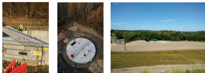
▲ Half way across ▲ Lift completed ▲ Site cleared
