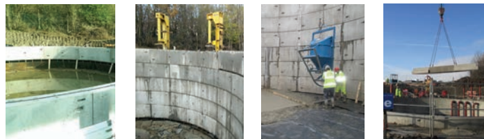
▲ Pre collar pour ▲ Placing segments ▲ Placing blinding ▲ First piece lifted
