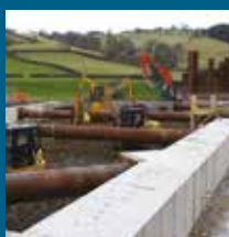
▲ Ring beam completed with struts in place
