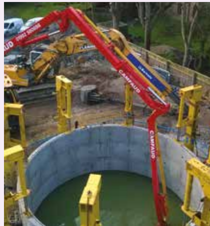
▲ Pumping of the plug to the 7.5m diameter 13m deep storage shaft
