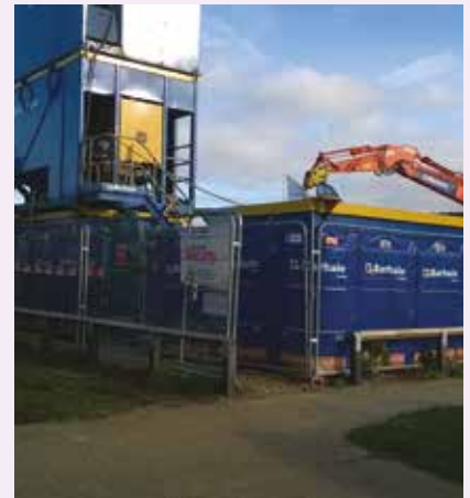
▲ The site office entrance with the tunnelling mud separation plant stack and a machine servicing the tunnel drive. The Herras fence is bounded by soundproofing barriers to prevent an environmental nuisance to the immediately adjacent residential properties.
