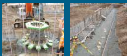
▲ Munching piles using a hydraulic pile breaker
