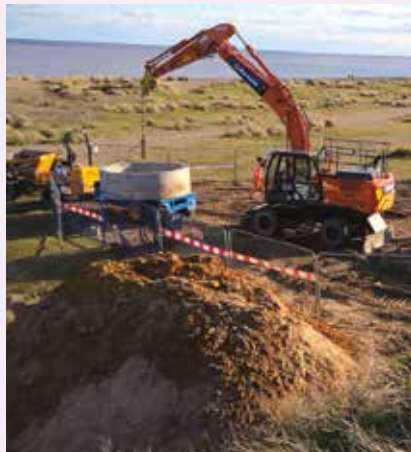
▲ The shaft above is the reception for the 600mm diameter sewer, which will soak away onto Pakefield beach. This sewer is surface water only so will just carry overflow from the existing network as well as 10 newly installed and connected road gullies.
