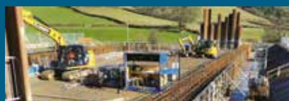
▲ Reinforcement being fixed for Ring Beam
