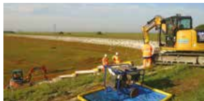
▲ Staines North Reservoir Maintenance Works
