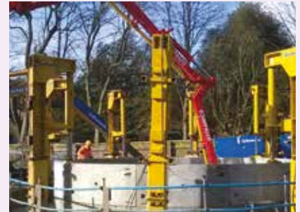
▲ Pumping of the plug to the 7.5m diameter 13m deep storage shaft
