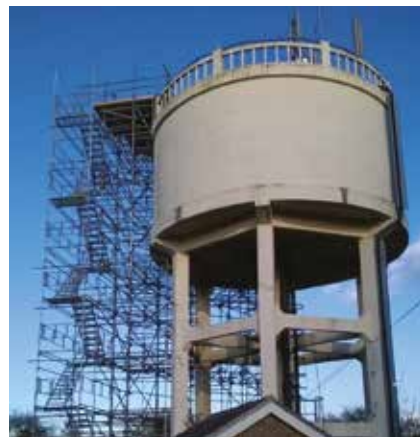
▲ Gazeley Water Tower
