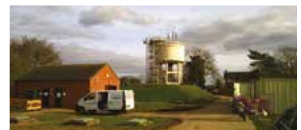
▲ Gazeley Water Tower
