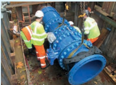
▲ Pipe installation at Horseguards Avenue
