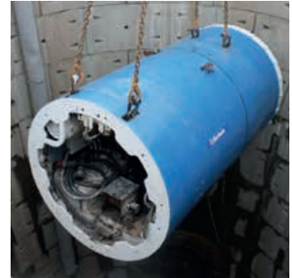
▲ Tunnel Boring Machine in shaft.
