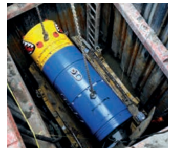
▲ Diglet being lowered into the ground.
