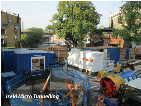
Shaft Construction
