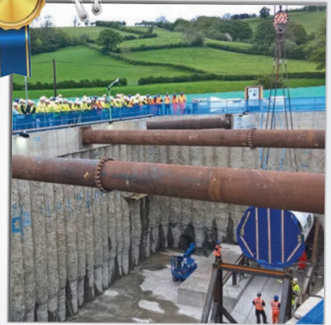
TBM launch on the Elan Valley Aqueduct Scheme Submitted by Roberto Sanchez Galan
