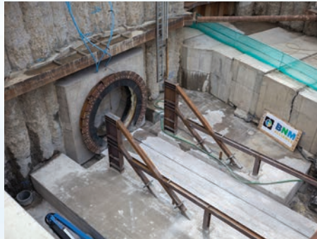
45m long x 25m wide drive pit
