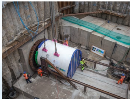
3m diameter TBM in position in drive pit
