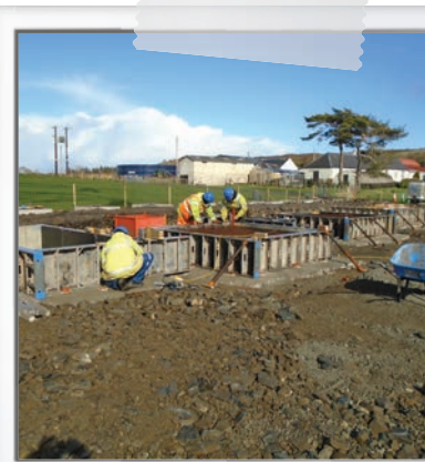
May runner up Chipperlaigen substation for Submitted by SPEN, Michal Hermanowicz
