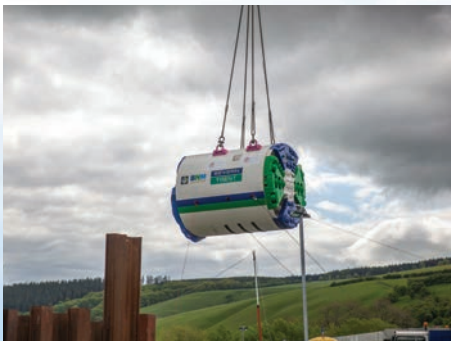
3m diameter TBM being lifted into the pit
