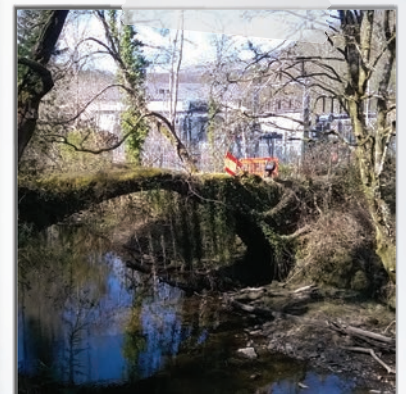
April runner up Maentwrog substation for SPEN Submitted by Colin Macken
