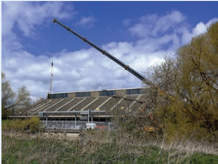
The entire 60m X 30m roof was refurbished
