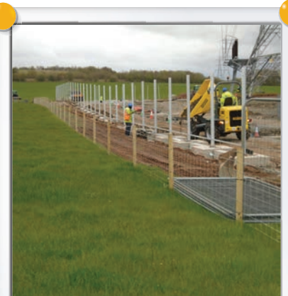
May runner up Chipperlaigen substation for Submitted by SPEN, Michal Hermanowicz
