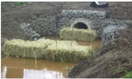
Straw bales to restrict flow from outfall
