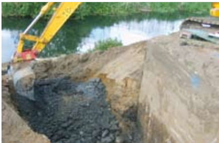
Digging out contaminated soil and inserting clay
