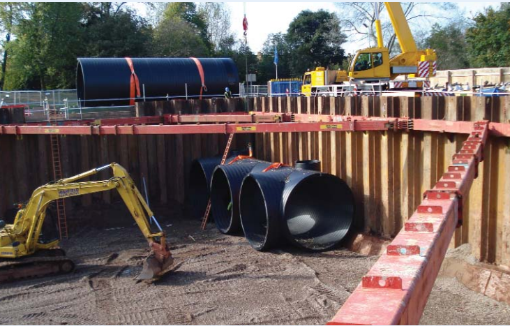
Barhale installs the Weholite storage pipes.
