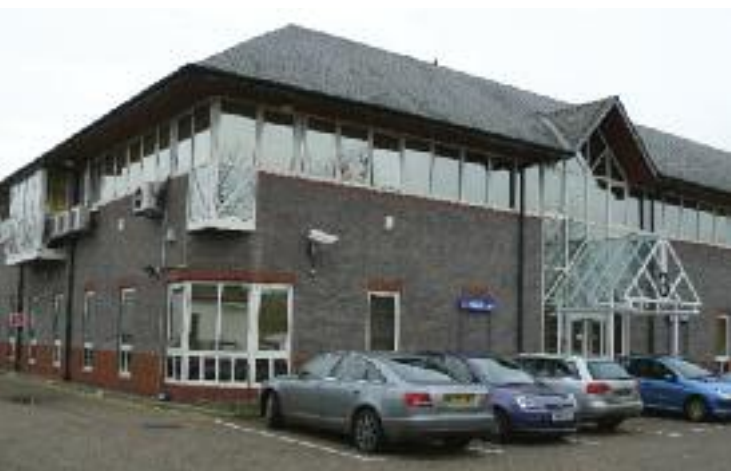
Southern Region's new Watford offices, above and right.
