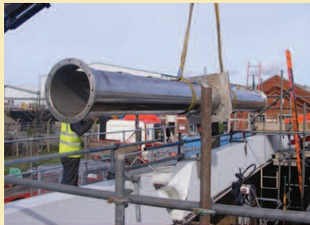
The PST de-scum device is lowered into position
